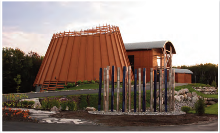
Built to honour the 400 th anniversary of the founding of Québec City, the Hôtel-Musée des Premières Nations in Wendake features an impressive architectural design and beautiful setting on the banks of the Saint-Charles River.
