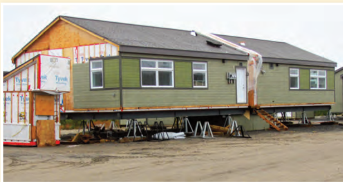
Semidetached homes under construction in Kuujuaq, 2010.
